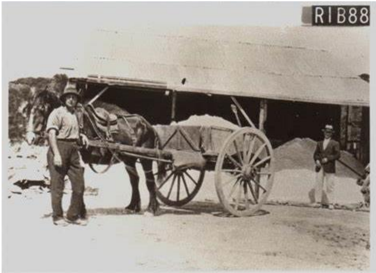
Figure 9 Photograph showing the salt store (RIB88).
