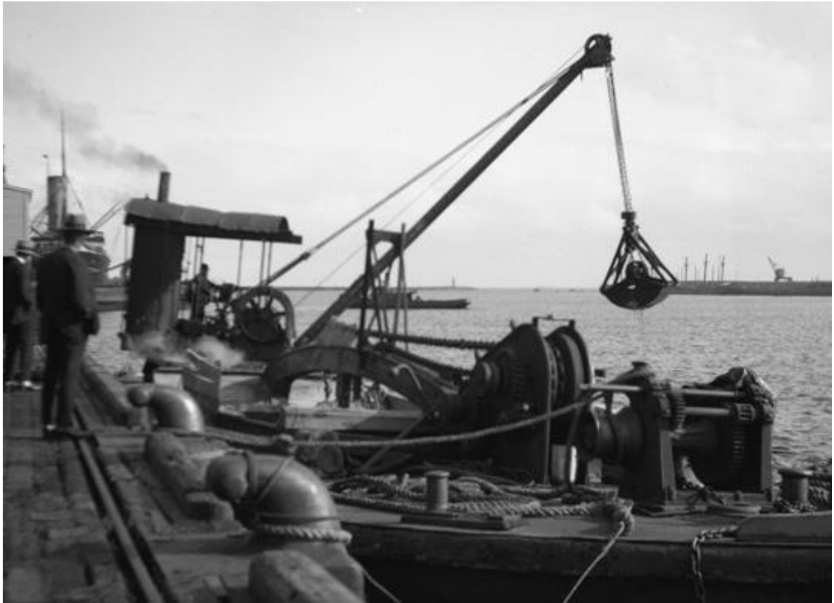
Figure 22 Steam powered Grab Crane Dredge operating in Fremantle Harbour 1924 (State Library of Western Australia).
