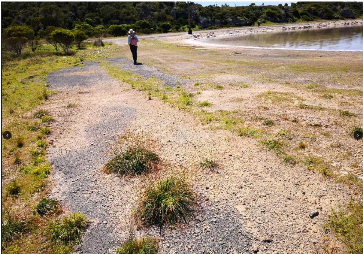
Figure 12 Salt_Store_020 – metaled road surface.
