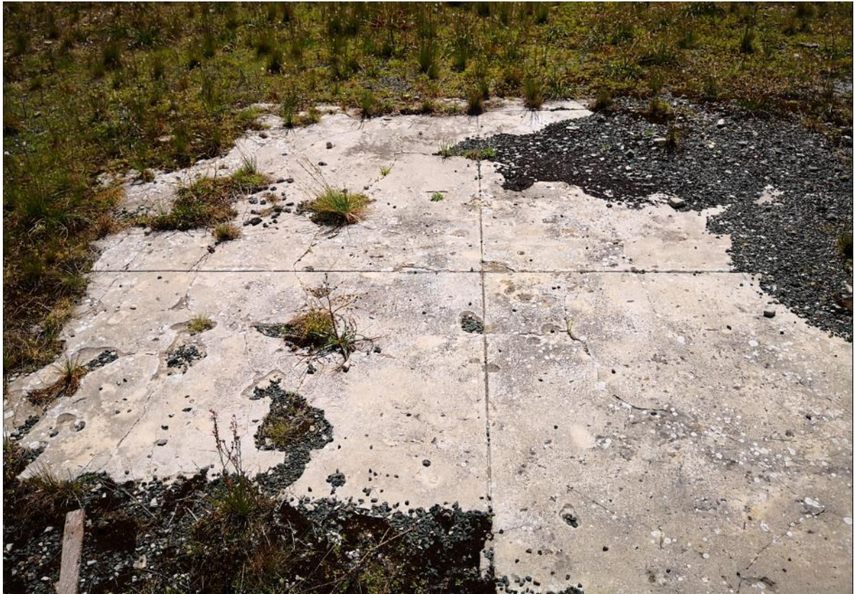
Figure 11 Salt_Store_019 – concrete surface to western side of salt store.
